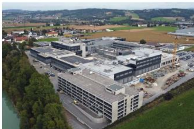
Figure 3: Aerial view of EV Group's corporate headquarters in St. Florian, Austria. In the foreground are the completed Manufacturing IV and V buildings, as well as the Manufacturing VI building, which is under construction.
