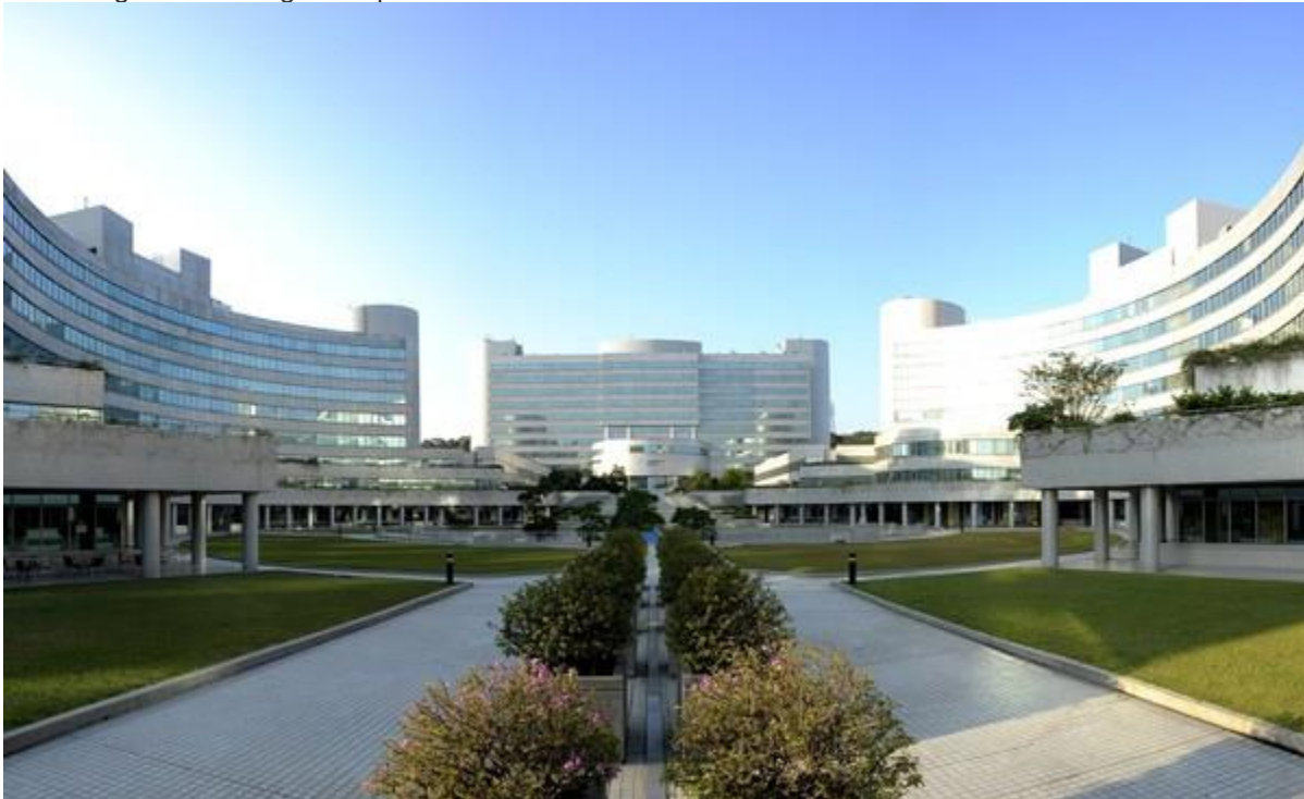
ITRI Headquarters, Chutung, Hsinchu County, Taiwan. Source: ITRI.
